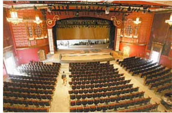
NANCEE E. LEWIS / Union-Tribune Architect Steve Bundy, son of project architect Richard Bundy, checked the reinstallation of the remaining original seats in the auditorium.
